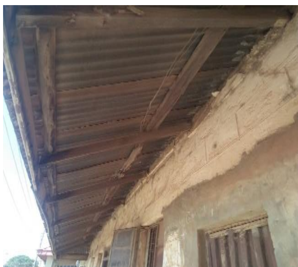
Plate X: Showing roof eaves without ceiling material.
